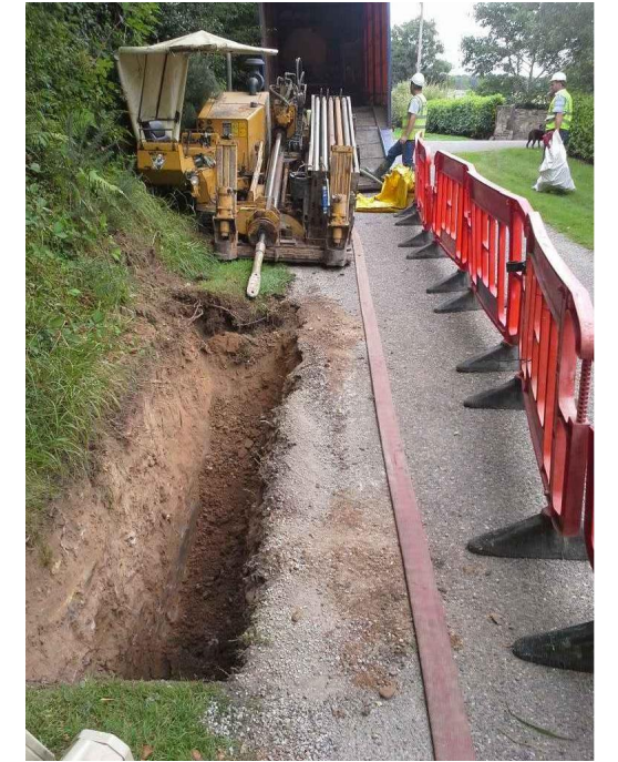
Image 2 : Typical Drilling Rig and Launch Pit
